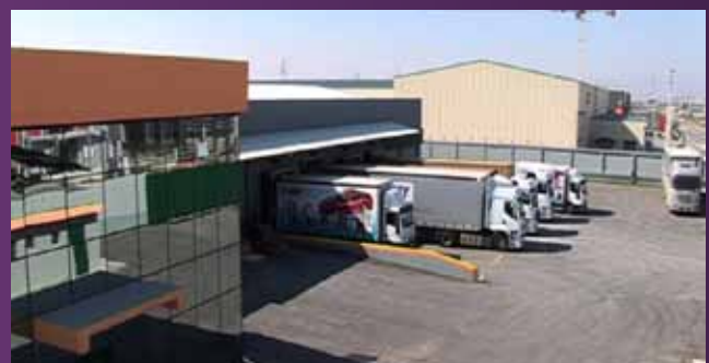
Distribution centre (11.000m 2 )
